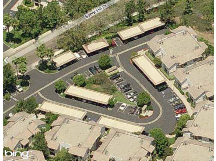
Figure 18 - Aerial Photo of a Multi-Unit Dwelling show several physical barriers to charger installation
